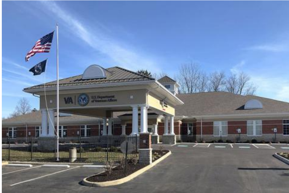
Springfield VA Clinic located in Springfield, Ohio. (VA Courtesy Photo)
